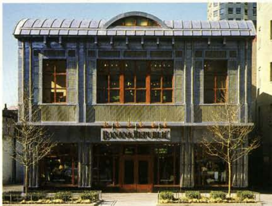
Above: A concrete structure along N. Michigan Avenue was turned into this barrel-vaulted facade of lead-coated copper reminiscent of the prefabricated metal structures exported to jungle colonies.
